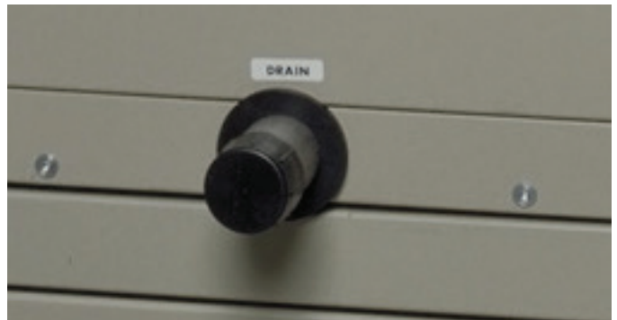
Figure 10: Coil Connections, Vents, Drains, and Drain Pan Connection, Extend Through Unit Cabinetry
